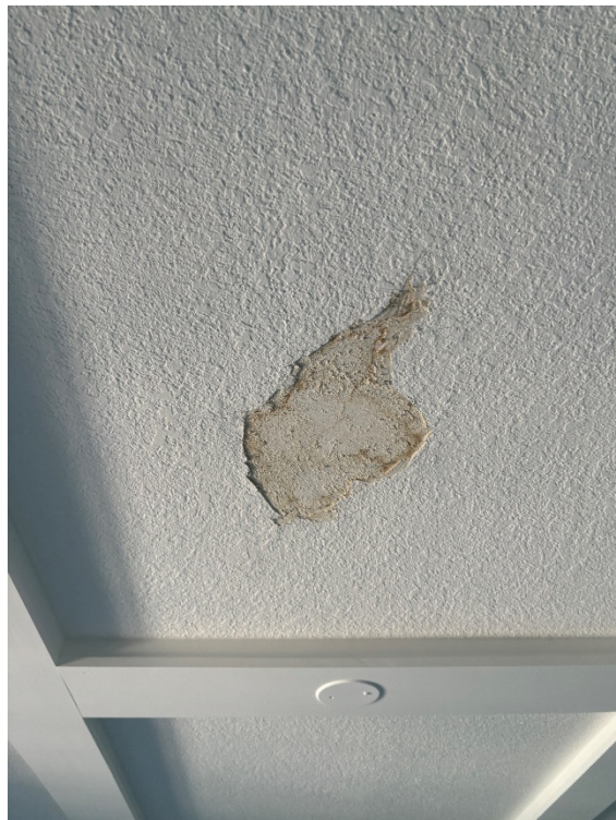
Water Damage in Ceiling of Master Bedroom Unit 602
