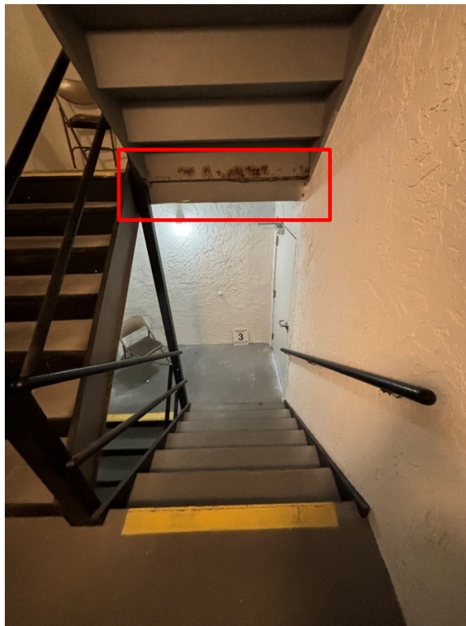
Deteriorating Concrete Steel Pan Identified in North Stairwell
