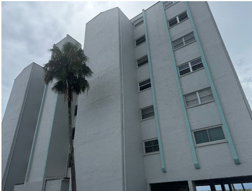
Rear Elevation of 403 Gulf Way
