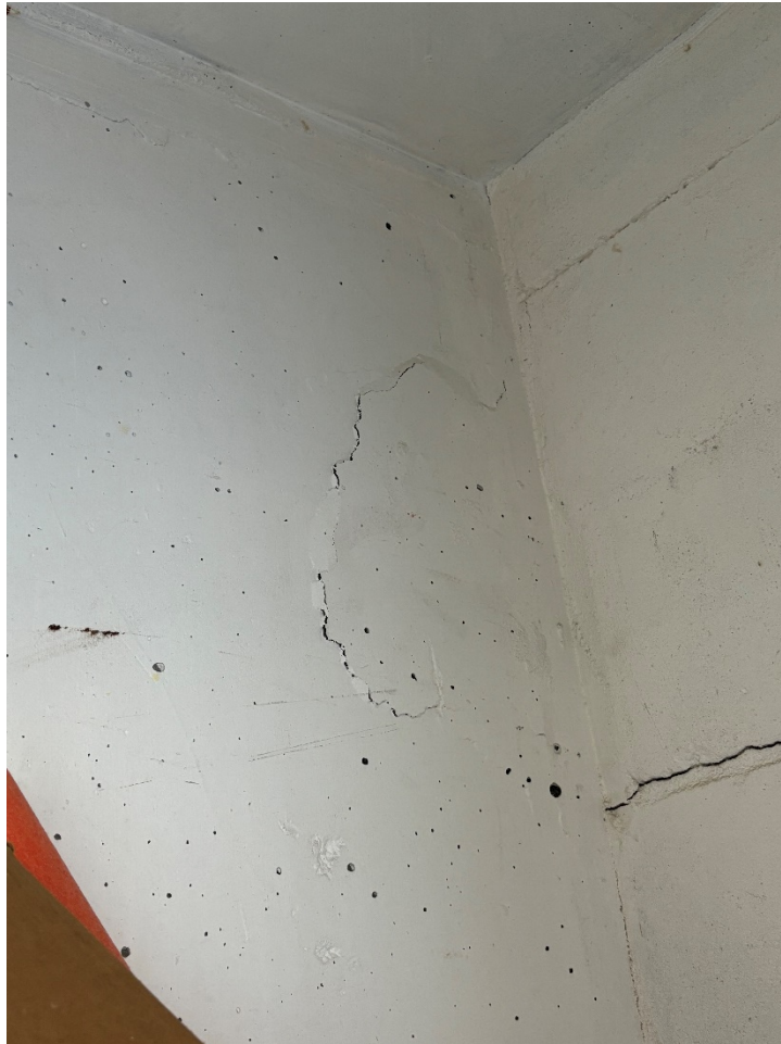
Isolated Spall to Concrete Column Unit 503 Balcony Closet
