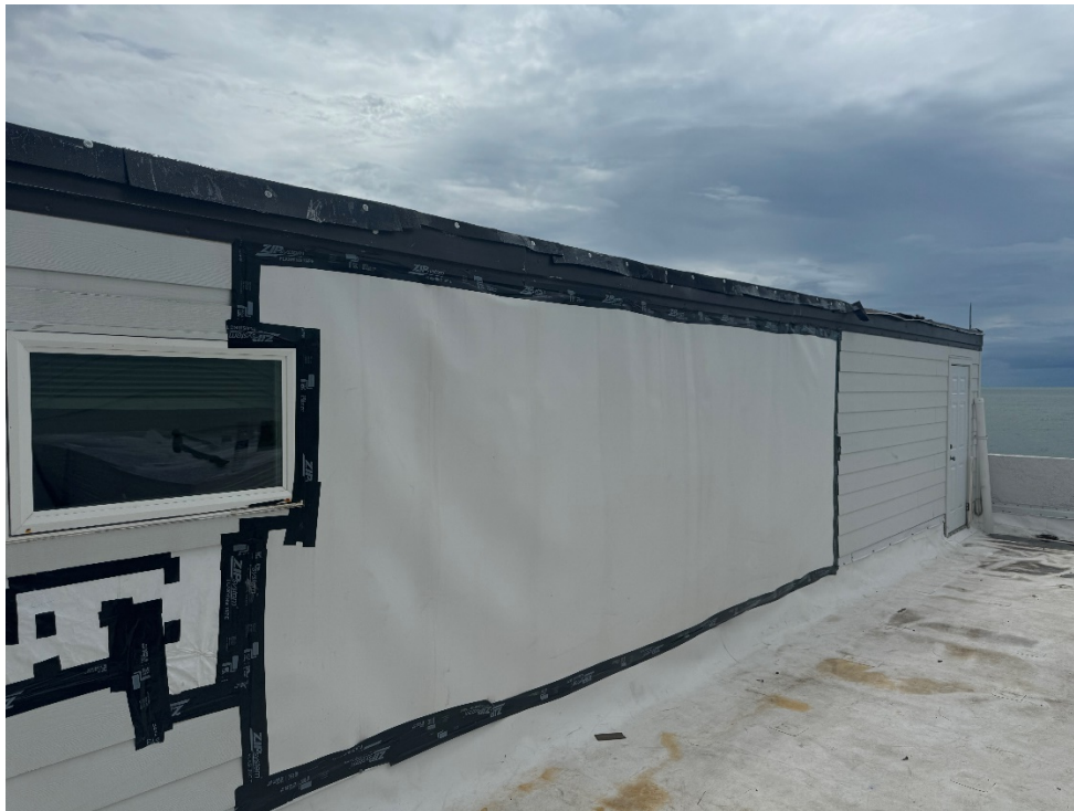
Exterior Frame Wall Reconstruction in Progress
