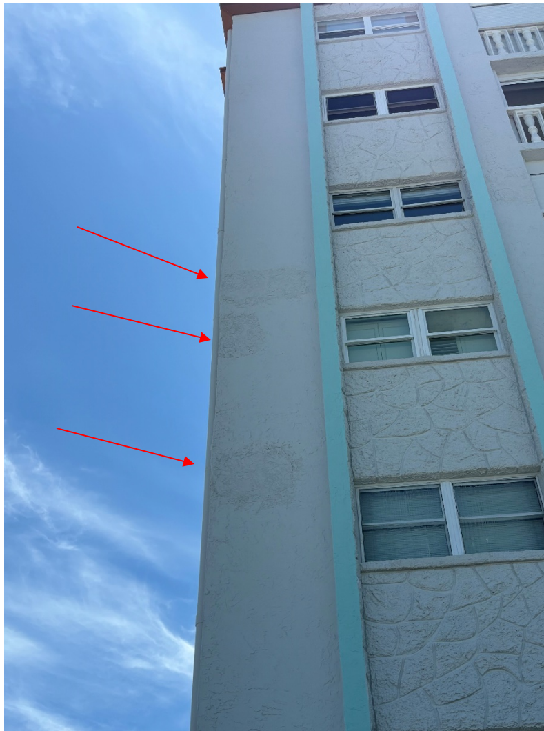
Stucco Repairs to Exterior Walls at Front Elevation of Building
