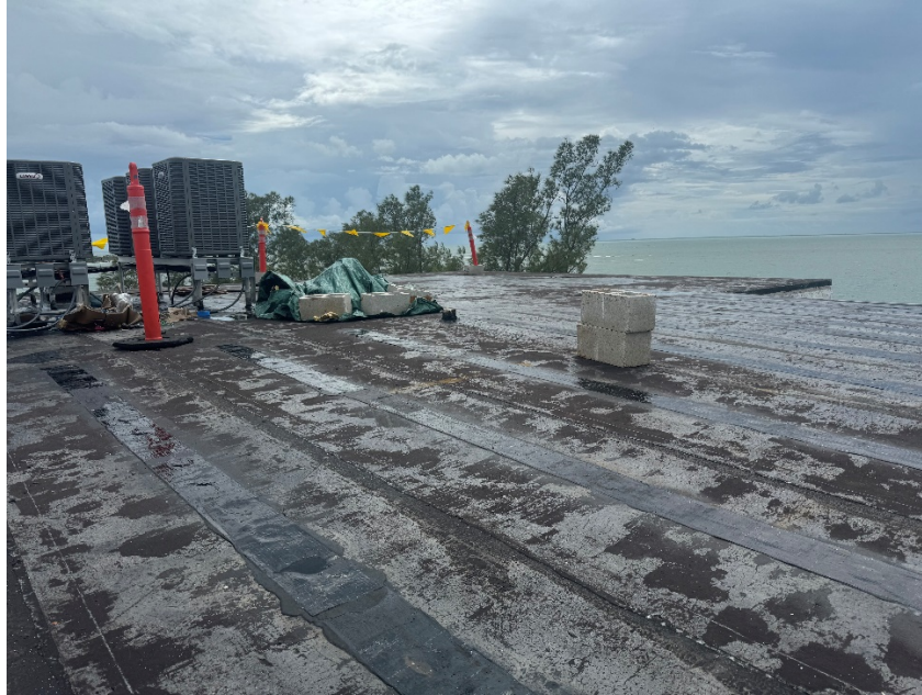
Roof Replacement in Progress with Dry-In Layer Currently in Place
