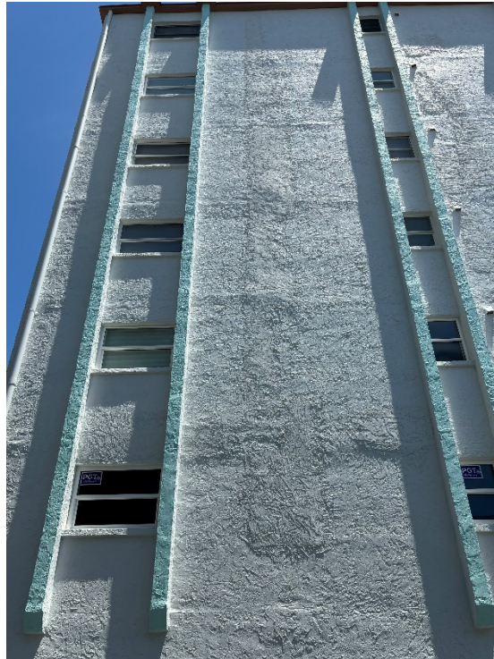
Stucco Repairs Visible at South Elevation of Building
