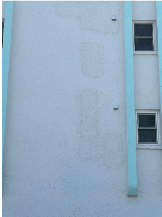
Stucco Repairs Visible at North Elevation of Building
