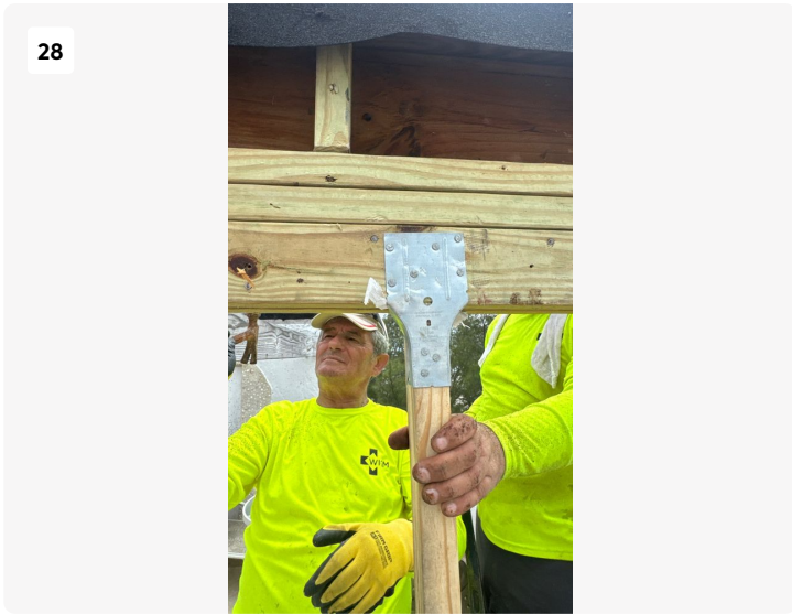
Framing repairs and hurricane clip installation.
